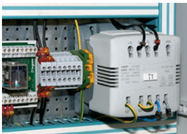
^ Supply of the auxiliaries adapted to the voltage and power requirements with Legrand control and signalling transformers
