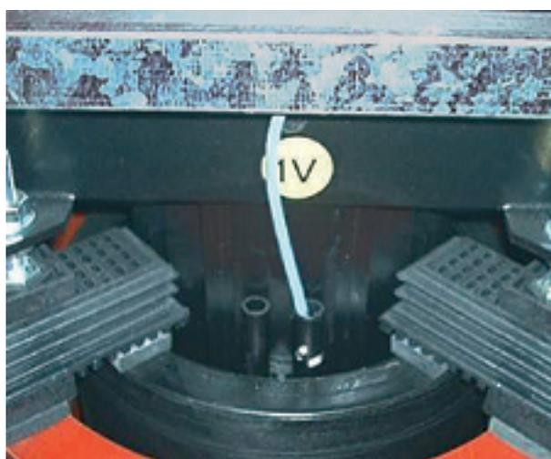
^ PCT sensor to check the temperature
