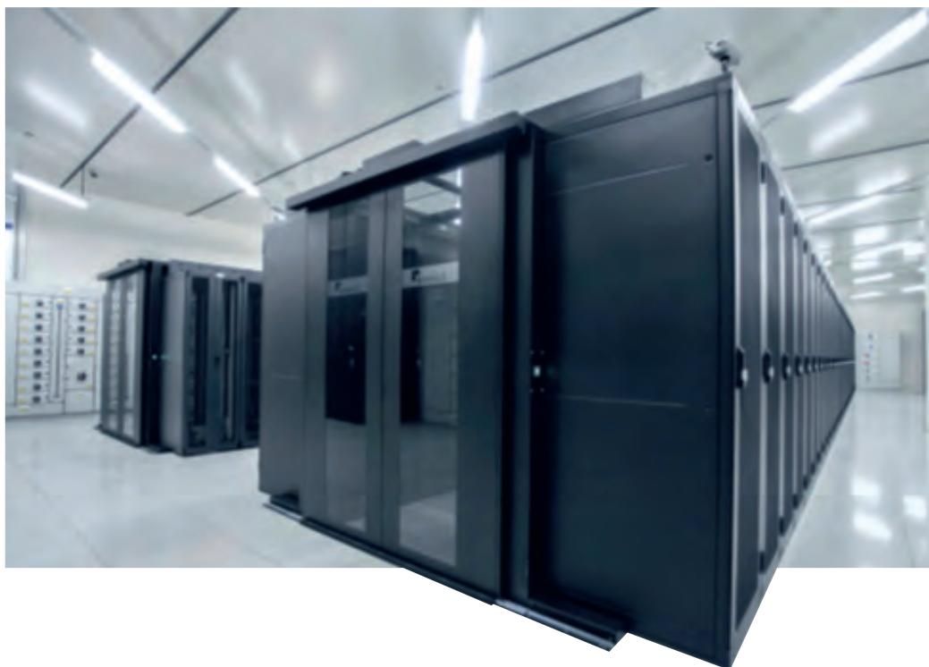
Modular data center
