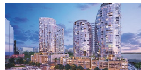
Location: Perth (Australia) Project: Ritz - Carlton Perth Legrand solutions: MSB / DBs / Meter Panels, Busbars, Arteor, Cablofil, Bticino Intercom (IP)
